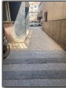
Figure (8) Detectable indicators, ramps and exterior handrails. Source: the researcher 2023.
